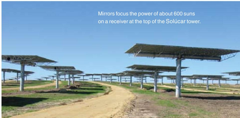
Mirrors focus the power of about 600 suns on a receiver at the top of the Solúcar tower.
